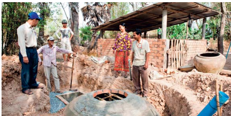
Installation of a biogas unit (credit EcoAct- SNV).
