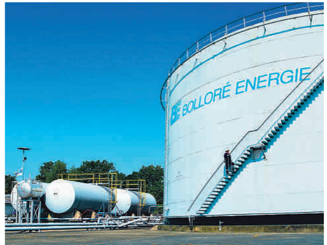
Tank, Strasbourg – France.
